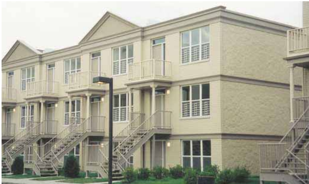
Affordable Concepts Inc. has expanded on its use of precast concrete wall panels for single-family homes with a new development featuring row houses. The houses feature a demising wall between units but otherwise feature the same design as some of the company's other single-family units.
