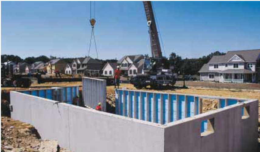
Insulated precast wall panels are being used in many states as foundation walls. The precaster who franchises this concept now is looking to use the panels as façades in key coastal states where durability is a prime consideration.
