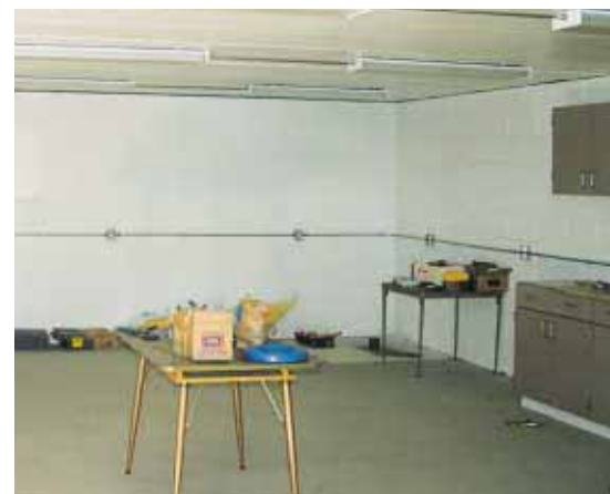
(Left) Only a few hollowcore slabs are required to span a new room under the garage, completing the process quickly.
